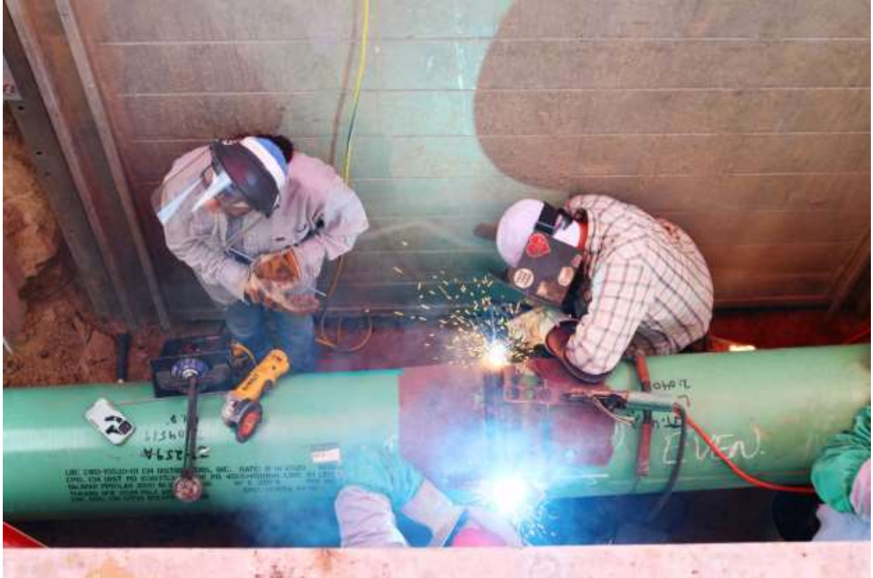
Crews working for SDG&E welding newly installed pipe along Pomerado Road north of Stone Canyon Road
